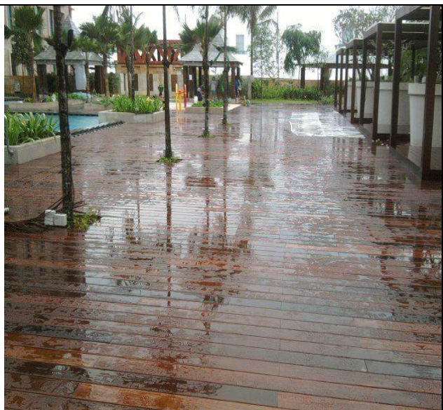
Ironwood Decking at Festive Hotel Sentosa
