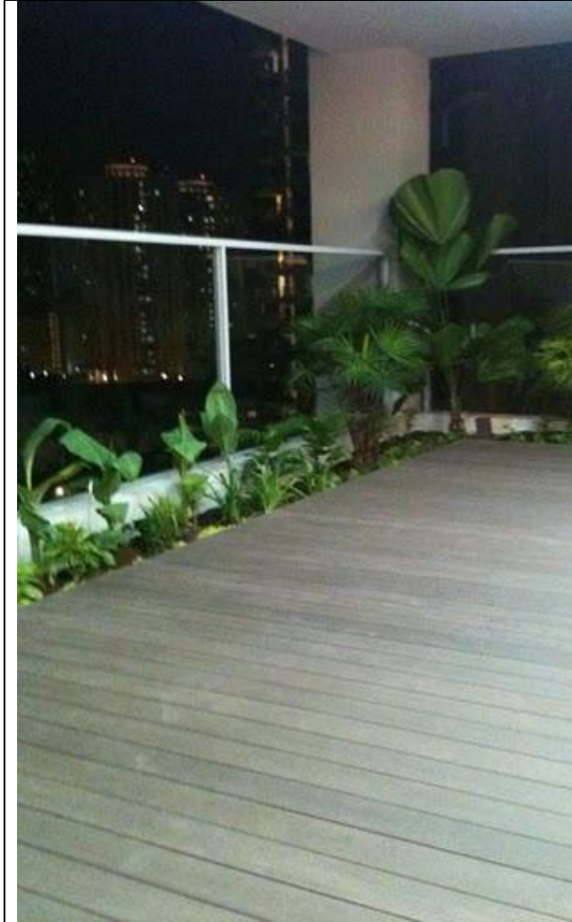
Composite decking at a Condo Public Area
